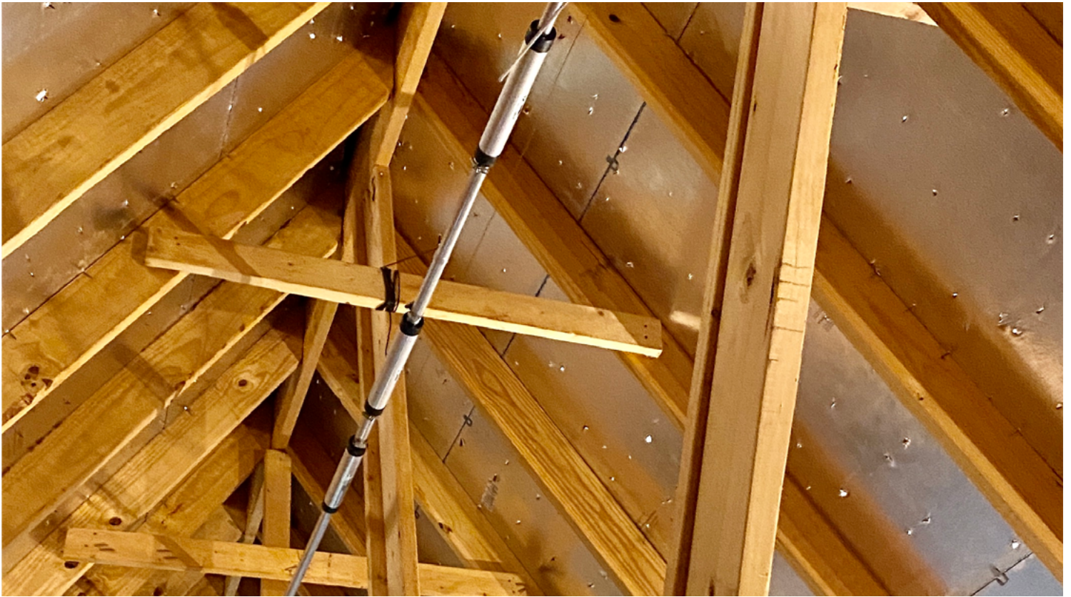
Cushcraft D4 rotatable dipole mounted in the author's attic space. OK, there's no rotating this dipole so who will hear these signals and will the foil-back insulating panels block the signals? (K4FMH photo)
