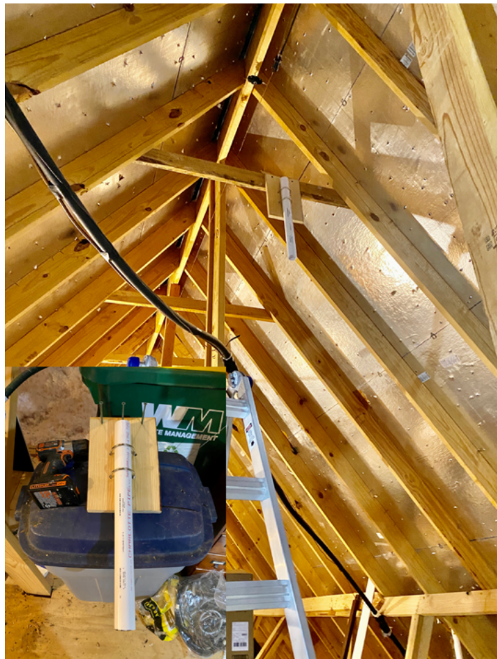
Final Mount of Cushcraft D4 (note paracord string and capacity hats)
